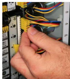
Relay #43 connection to fourth relay module
